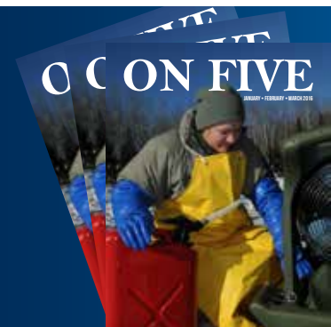
Airman 1st Class Hannah Race, 148th Fighter Wing Communications Flight, checks the fuel level of a generator Feb. 2, 2016. Eight Communication's Flight Airmen were at a remote site approximately seven miles from Grand Marais, Minn., supporting the John Beargrease Sled Dog Race and training in cold weather conditions. (U.S. Air National Guard photo by Master Sgt. Ralph Kapustka)
