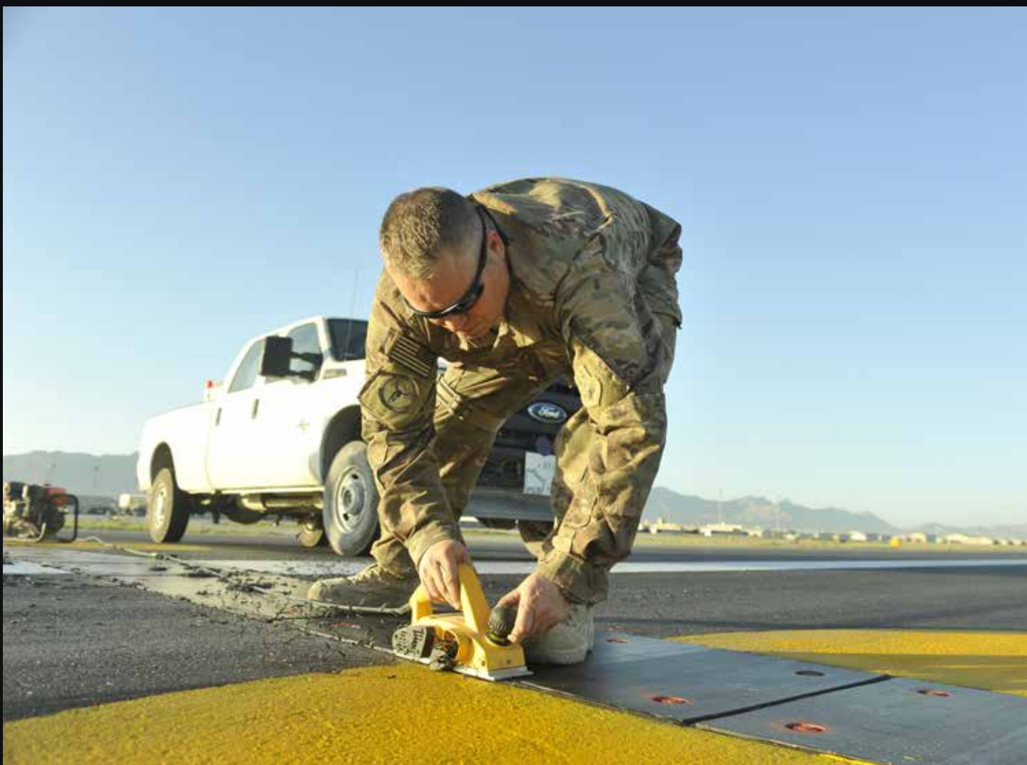
Senior Master Sgt. Douglas Ion, 455th Expeditionary Civil Engineer Squadron project non-commissioned officer in charge, uses a power planer to remove poly panel material to prevent potential aircraft mishaps on the flightline at Bagram Airfield, Afghanistan June 9th, 2014. Ion is a native of Duluth, Minnesota and is deployed from the Air National Guards' 148th Fighter Wing, Duluth, Minnesota. (U.S. Air Force photo by Airman 1st Class Bobby Cummings)
